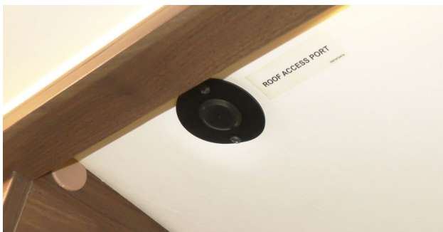
Roof Access Port (Located inside the passenger front overhead) -Typical View
