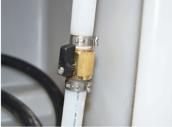
Water Tank Drain Valve -Typical installation shown
