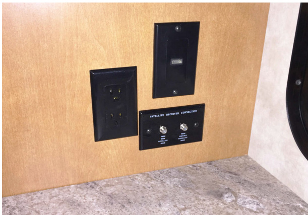
Bedroom DVD/Satellite Receiver Connection -Typical View
